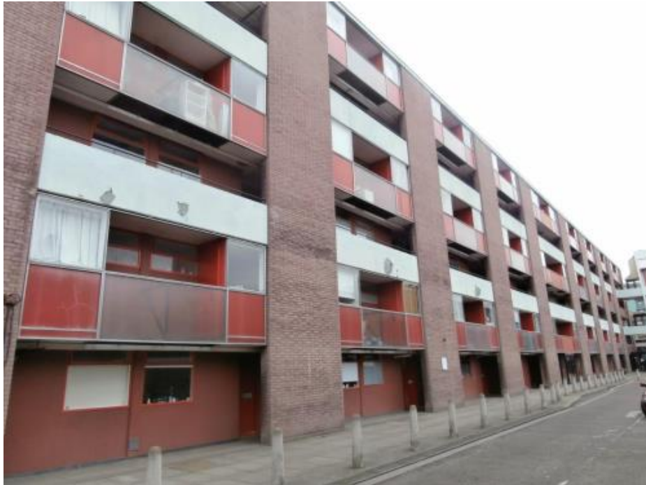
Basterfield House northern elevation
